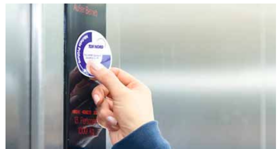
The inspection sticker shows the scheduled date of the next lift test.
