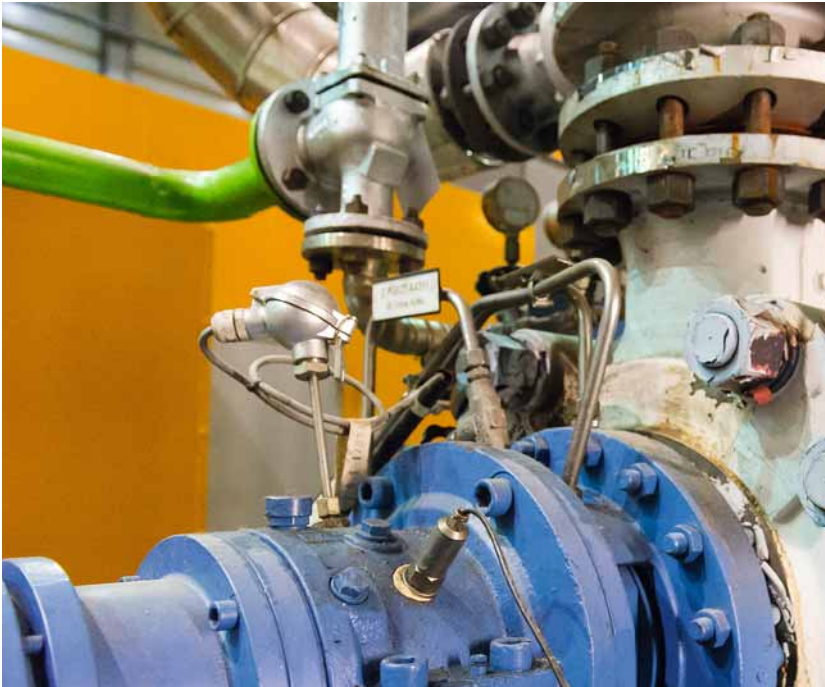
Structure-borne-sound sensors measure the functioning of the structural units in the harsh refinery environment and transmit the data to the server.
