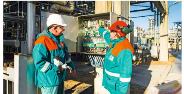
The Wi-Fi detection unit from DMT in the refinery is inspected by Dr Thomas Leyh (left) and Matthias Harms.
