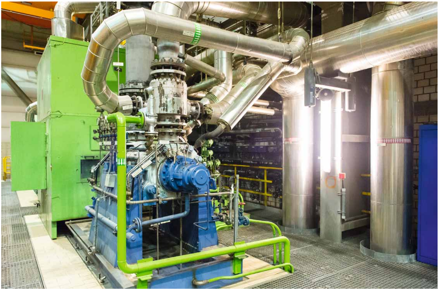
The feed pump unit in the industrial power plant of the PCK Raffinerie is under constant surveillance.
