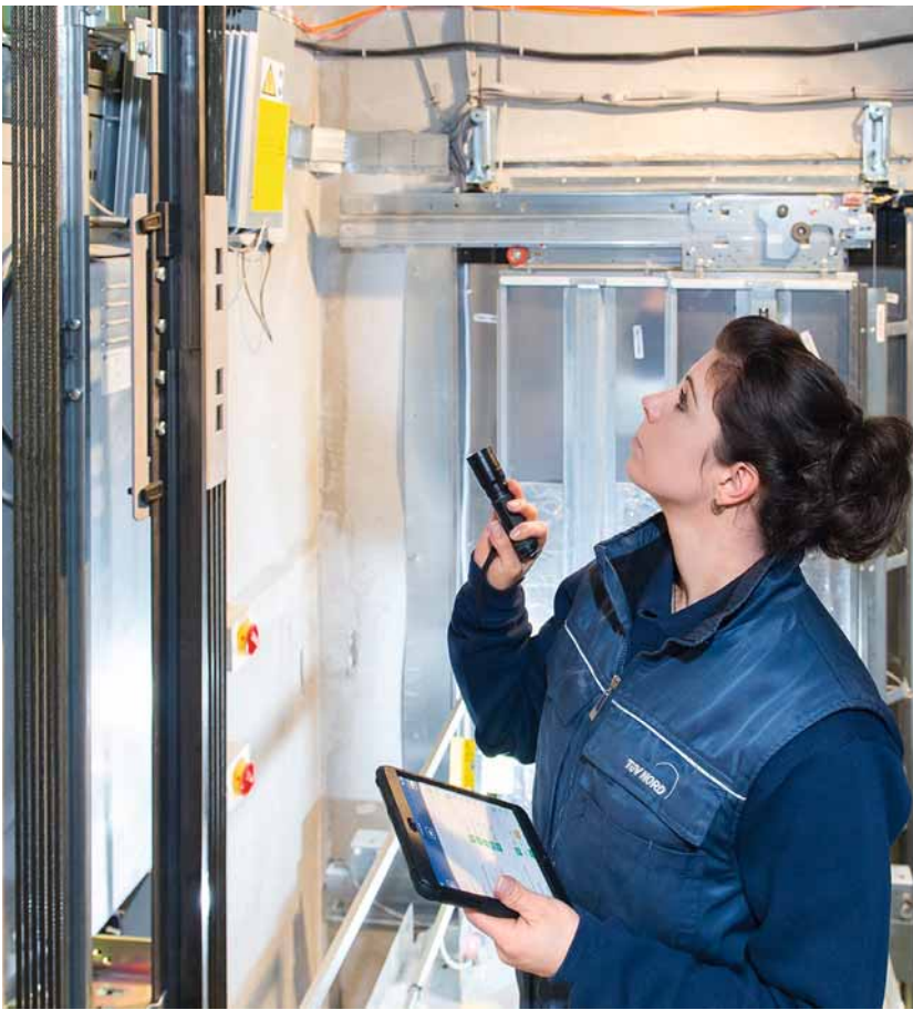
In the lift shaft, the testers check components such as the drive gear, brake and doors.
